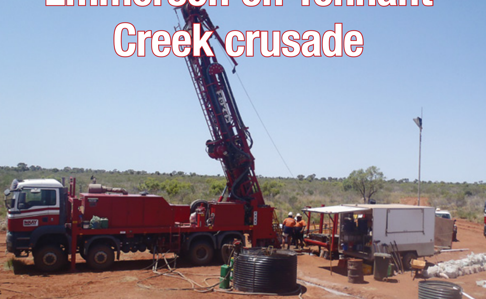
Drilling on Emmerson Resources Ltd's Red Bluff project in Tennant Creek. Thanks to its JV with Ivanhoe Australia Ltd Emmerson is managing $9 million of drilling each year for the next three years
