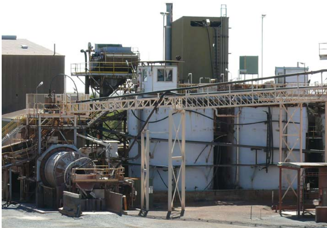
The Warrego milling complex is one of the company's key strategic assets.
